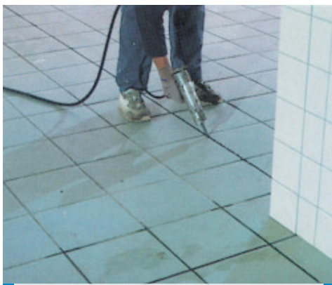
Sealing ceramic tile floor with Mapesil AC
