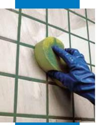
Cleaning and finishing the tile joints on a wall with a sponge
