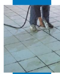
Sealing ceramic tile floor with Mapesil AC
