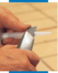
Cutting the nozzle according to the size of the joints
