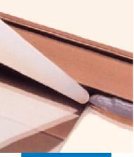
Sealing aluminium window frame with Mapesil AC
