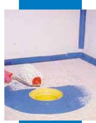
The special piece of Mapeband embedded in the Mapegum WPS
