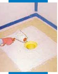
Spreading Mapegum WPS around the drain in a shower cubicle
