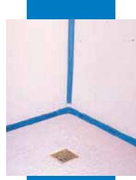
End result of a waterproofing treatment using Mapegum WPS and Mapeband
