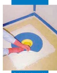
Positioning the special piece of Mapeband over Mapegum WPS
